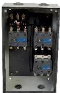
Interior View of ML SASD
