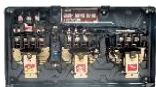
Interior View of MK1 FASD
